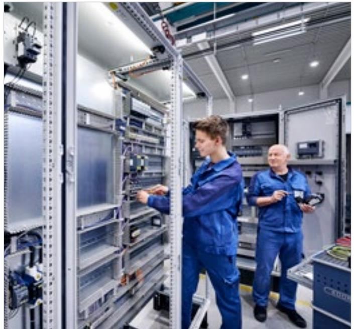
Example control cabinet with control system for either one or more Ploughshare® Mixers or for a complete mixing line with all system components (depending on customer requirements)
